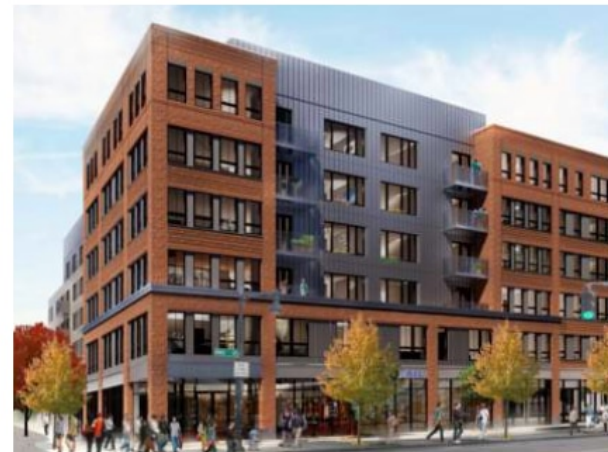
KENDALL EAST, CAMBRIDGE, MA Construction Costs: $54,000,000 Completion Date: Nov. 2021
