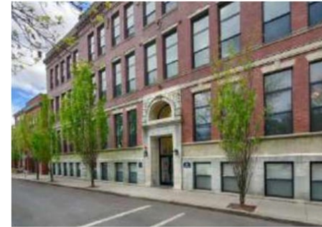
DANA PARK PLACE, CAMBRIDGE, MA Construction Costs: $7,800,000 Completion Date: Aug. 2010
