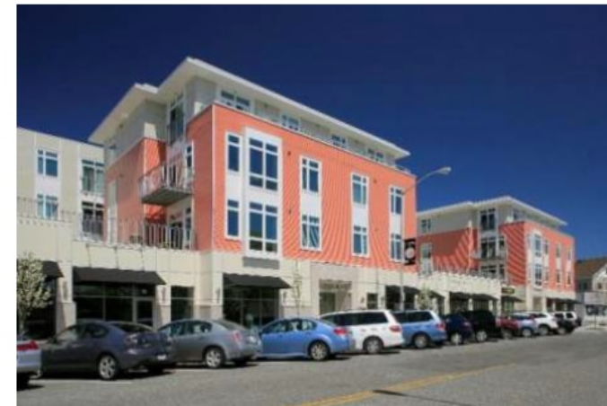
30 HAVEN, READING, MA Construction Costs: $12,700,000 Completion Date: Sept. 2012
