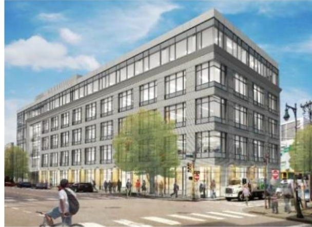
121 FIRST STREET, CAMBRIDGE, MA Construction Costs: $14,600,000 Completion Date: Sept. 2018
